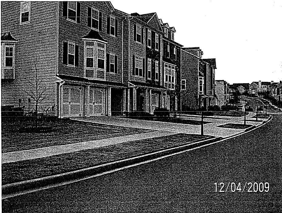
Existing Units along Park Pass Way in Unit IIA
