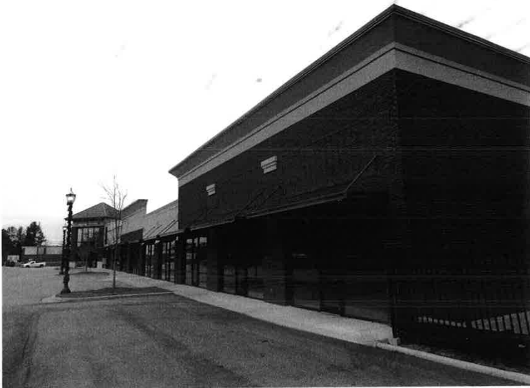
Photo 4: Southeast Elevation Detail- existing to remain unchanged
