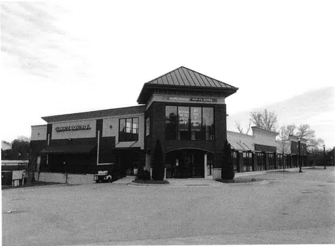
Photo 1: Southwest Elevation Overall- existing to remain unchanged
