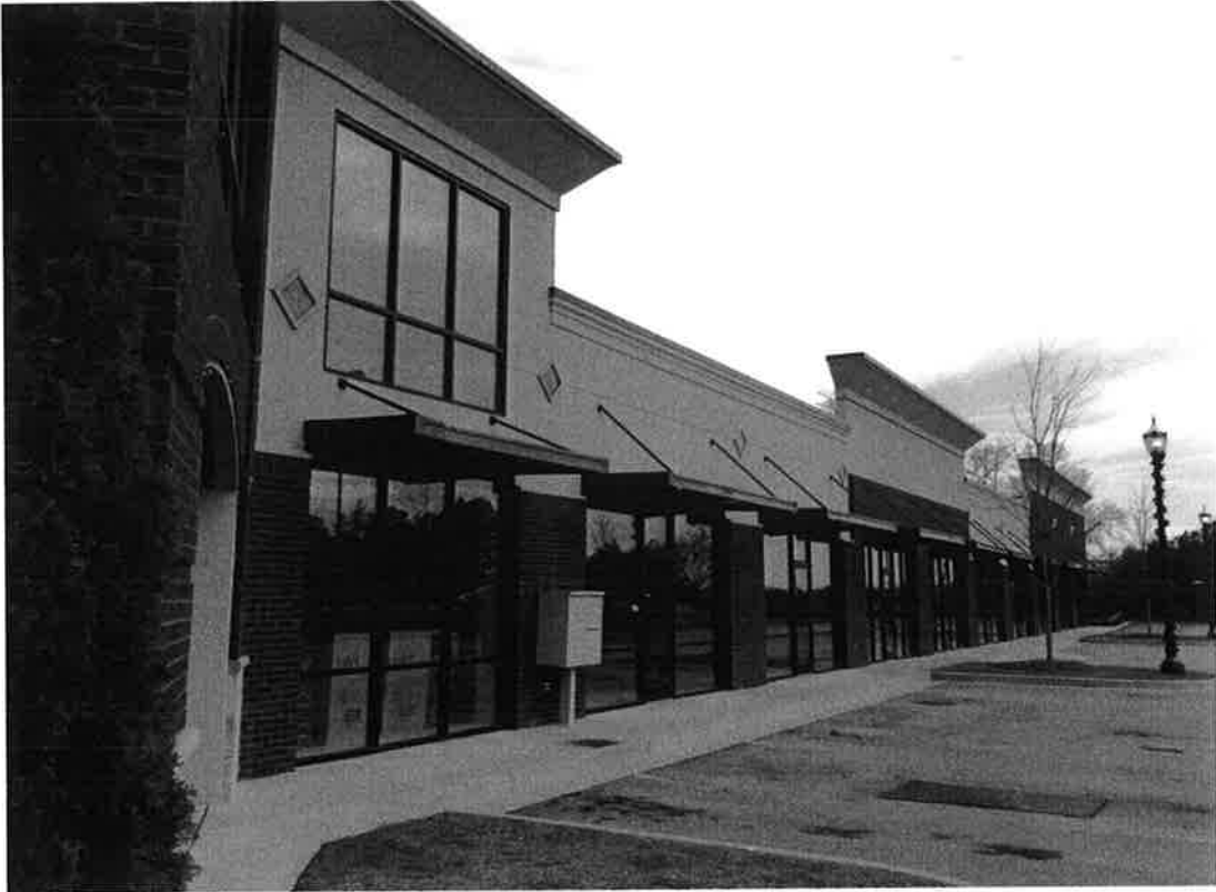
Photo 3: Southwest Elevation Detail- existing to remain unchanged
