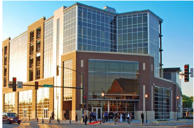
A performance space occupies the first floor of this mixed use building in downtown Coralville, Iowa (image courtesy City of Coralville)
