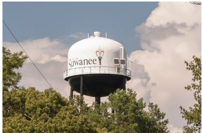
The City of Suwanee has invested considerable efforts to update its water system
