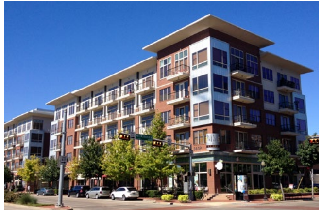
Mixed-use buildings will extend the sidewalk retail experience of Town Center as well as provide a large number of residents to make the area more vibrant
