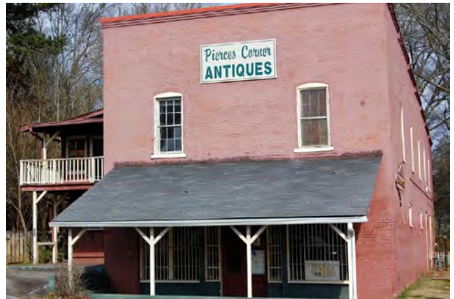
Pierce's Corner is a valuable historic resource in Old Town and is eligible for historic tax credits
