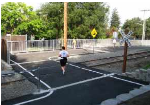
Trail railroad crossing in Seattle
